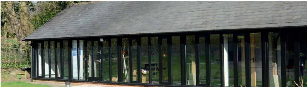
Example of a converted barn in Farleigh Road now being used as offices
