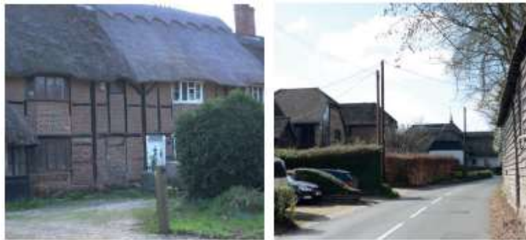
Farleigh Road thatch and barn
