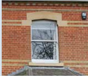
Sash window and fenestration detail
