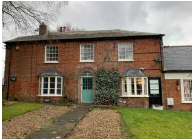
Figure 18: The Old bakery Emporium on Aldermaston Road, which features many positive Victorian details such as bay windows red clay tiles.
