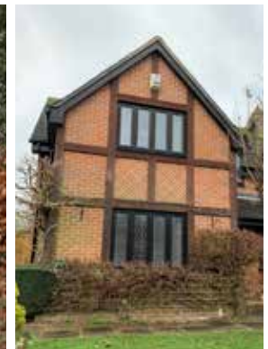
Figure 107: Red brick front, exposed timber frame
