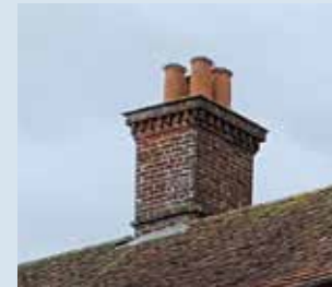
Masonry chimney stack
