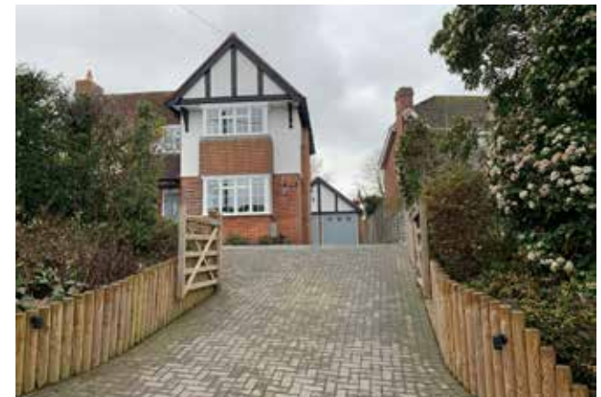
Figure 48: Wooden fencing and boundary planting, Elm Road, which forms a strong boundary and screens the elevated dwelling from the street.
