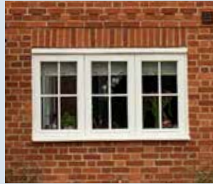
Window muntins and vertical brick details
