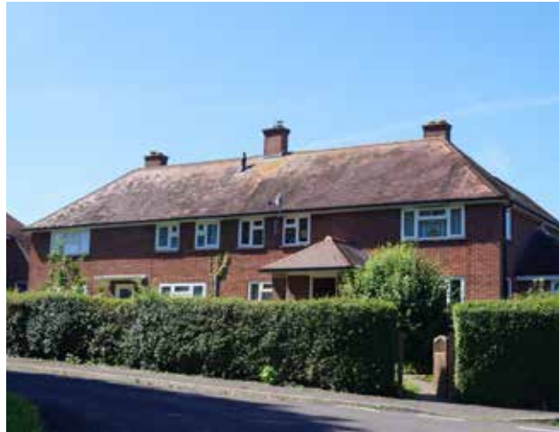
Figure 30: Semi-detached house which is typical to this CA with red brick and a tiled, hipped roof.
