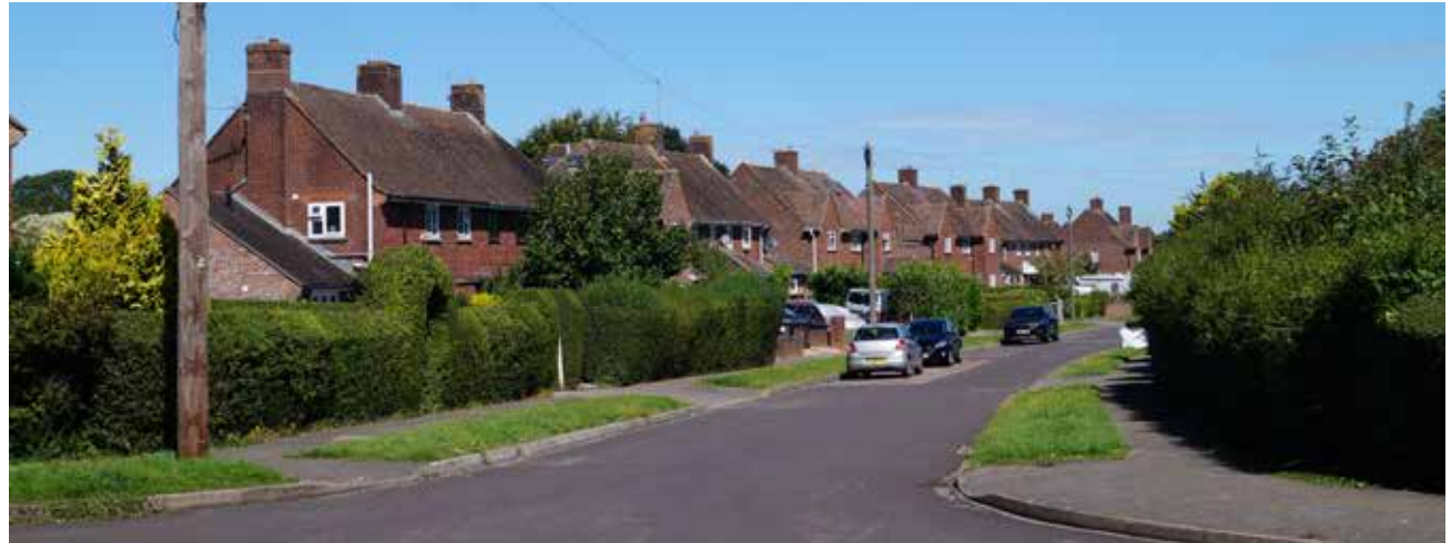
Figure 28: View of the two-storey brick houses from the entrance into the Spring Close cul-de-sac.
