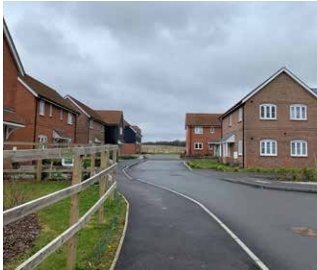
Figure 43: Detached houses, Sireburn Close with clay tile, red brick and timber weatherboarding, in keeping with the historic character of the CA and the village. However due to the small gaps between buildings, short set back distances and use of hard boundary treatments the development has an urban feel which does not fully reflect the rural, village character of Sherborne St John.
