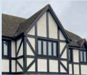
Exposed timber framework
