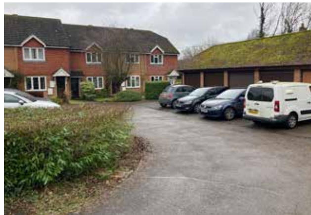
Figure 47: Terraced houses with courtyard parking, Cranesfield, which is somewhat out of character with the rest of the public realm in the village.
