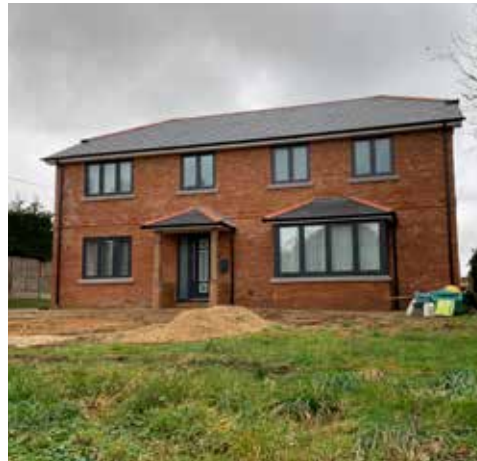
Figure 20: A modern detached house on Aldermaston Road, which reflects the historic material palette and architectural features, such as red brick, grey slate, bay windows and a porch.
